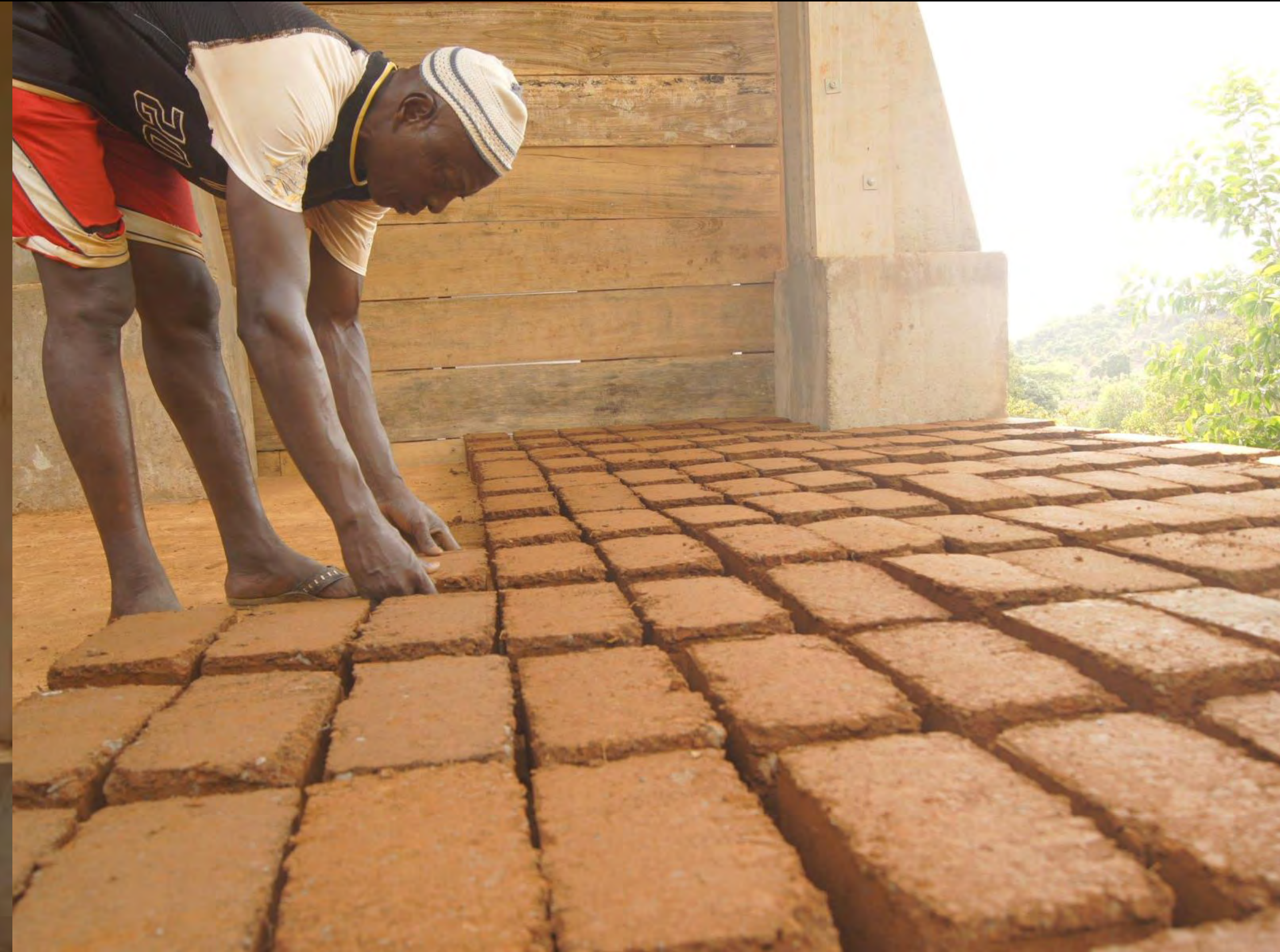
SOIL PRESS LOCAL SOIL PRESSED TO BRICKS
