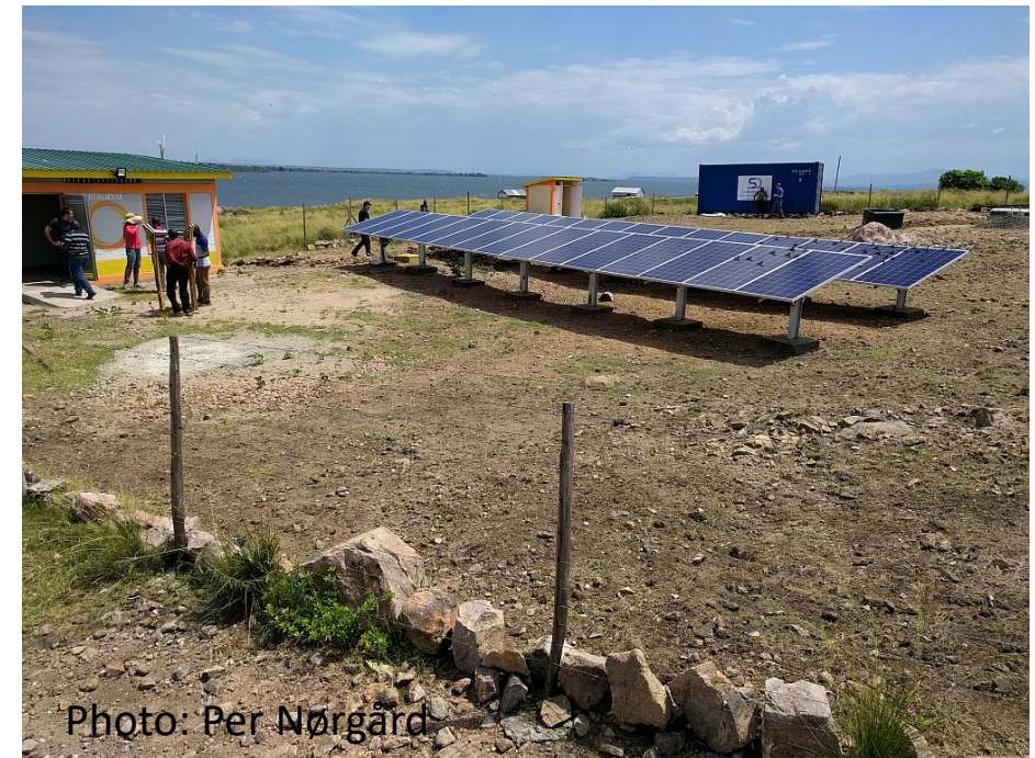
9 kW PV mini-grid on Ndeda island by Renewvia
